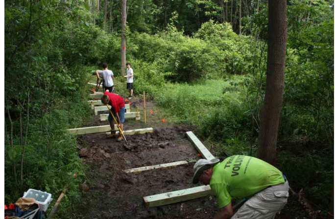
Laying down the foundation.
