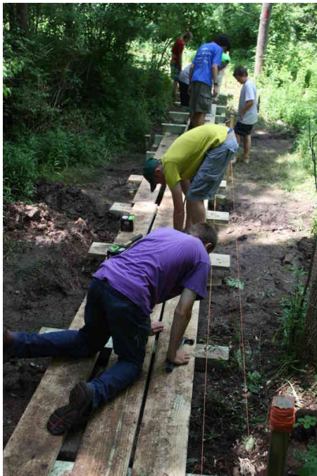
Nailing down the deck boards.
